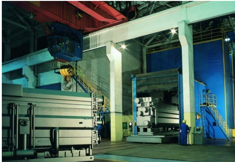
Whole Unit Shot-blasting
